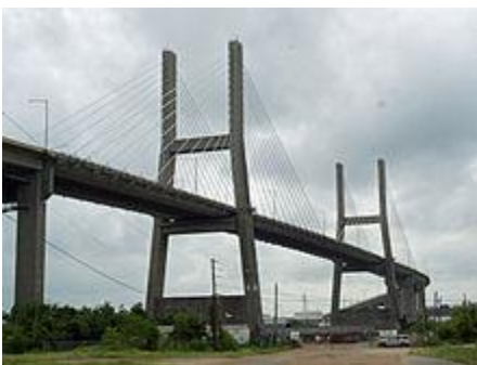
Today, Cochrane-Africatown Bridge on the northern side of Blakeley Island
