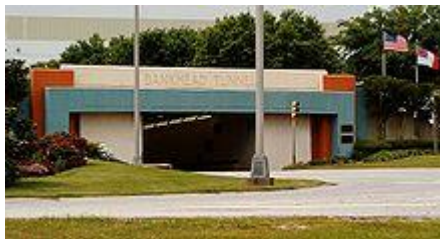
Today, eastern entrance of the Bankhead Tunnel on the southern side of Blakeley Island.
