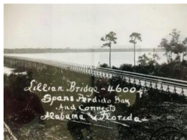
Old Lillian Bridge looking southeast
